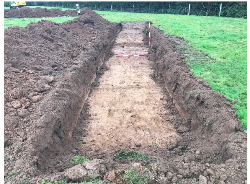
Plate 16: Test Trench 6, facing northeast
