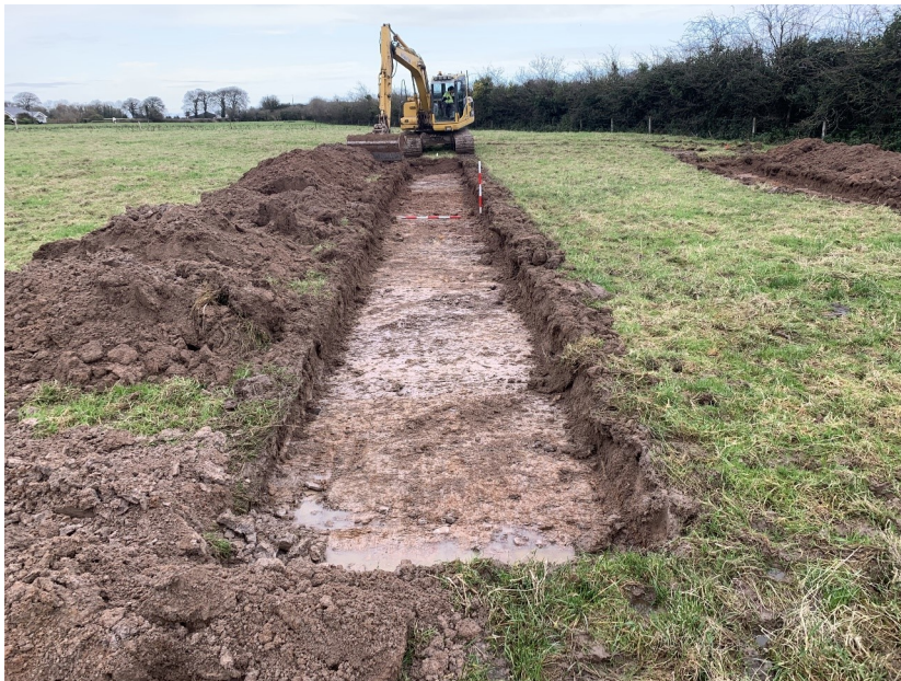
Plate 19: Test Trench 7, facing northeast
