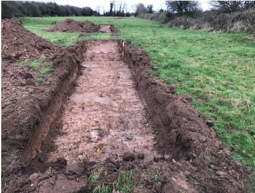
Plate 29: Test Trench 13, facing north
